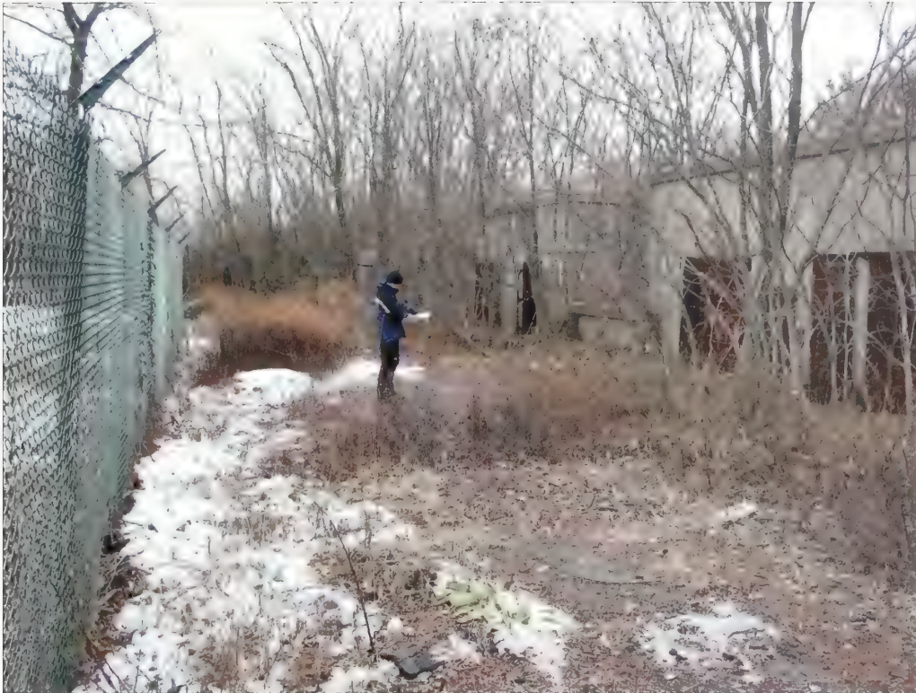
Figure 3.5. View looking west at U.S. Coast Guard perimeter fence and Battery Morris. There is currently no vehicular access to Battery Morris and staff and visitors wishing to see the structure walk on a trail surface comprised of broken asphalt and accumulated leaf litter and debris. Emerging woody vegetation obscures a clear definition of the trail and makes access difficult (Olmsted Center, January 2009).
